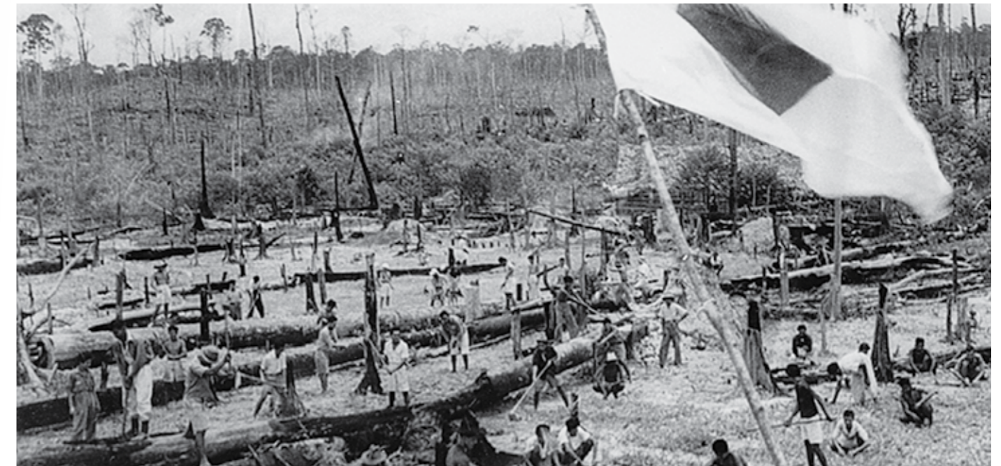
(Below) The first settlers to Bahau – mainly young, single men – had to clear the land, build a rudimentary road from the train station to the camp and set up basic infrastructure before the families started to arrive (Japanese propaganda photo). Courtesy of Father René Nicolas.
